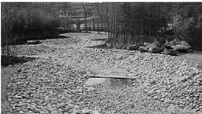
Figure 3-7. Construction of a meandering streambed covered with stones anchored in mortar (above), and after filling with water (above).
