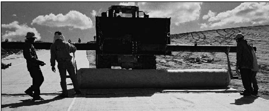
Figure 4-7. Typical means of liner deployment, using a backwards-moving front-end loader.
