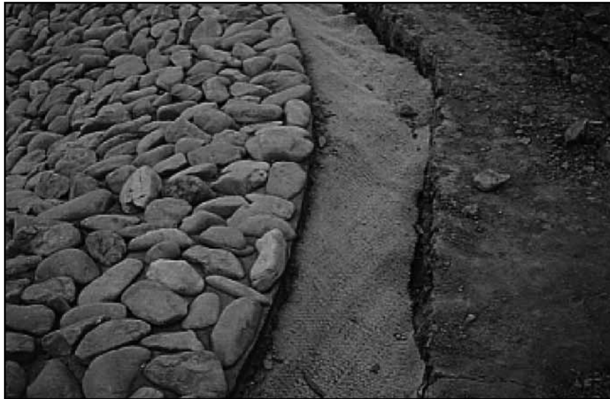
Figure 3-3. In this pond, a layer of cover soil protects the Bentomat CL and provides a foundation for a geotextile, upon which large stones are set in mortar. This armored slope will not be subject to erosion or deterioration by people or animals. This technique may not be applicable in freeze/thaw zones.
