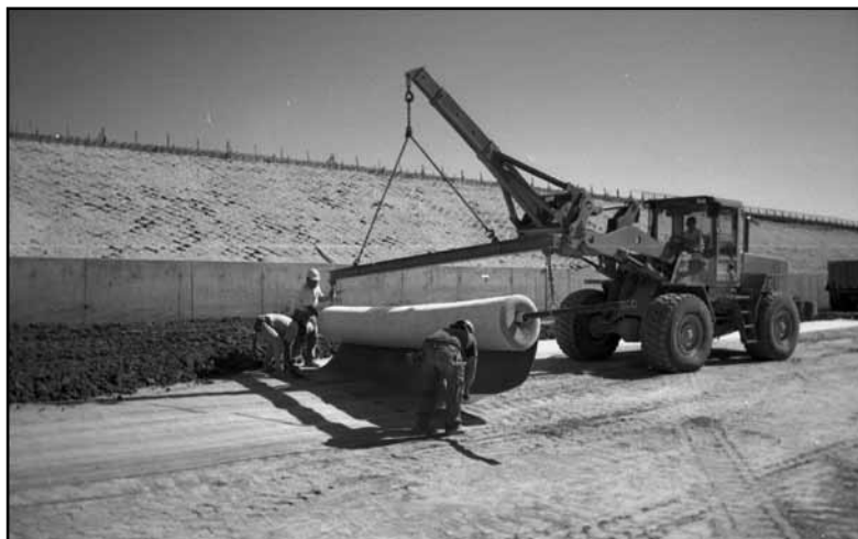
Figure 4-1. Deployment of the liner using core pipe and spreader bar.
