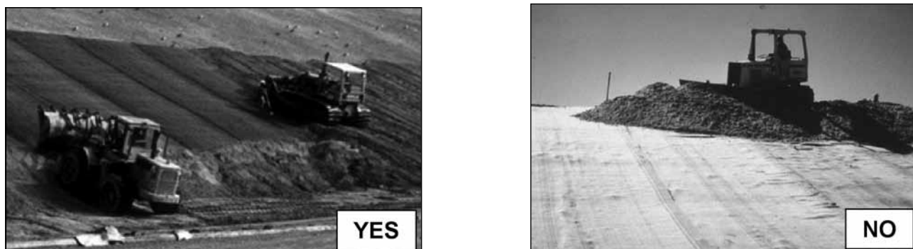
Figure 4-16. Cover soils should be pushed from the bottom of the slope up, not from the top down.
