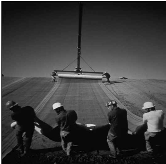
Figure 4-8. Manual deployment down a slope. It is generally not possible to pull the liner upslope.
