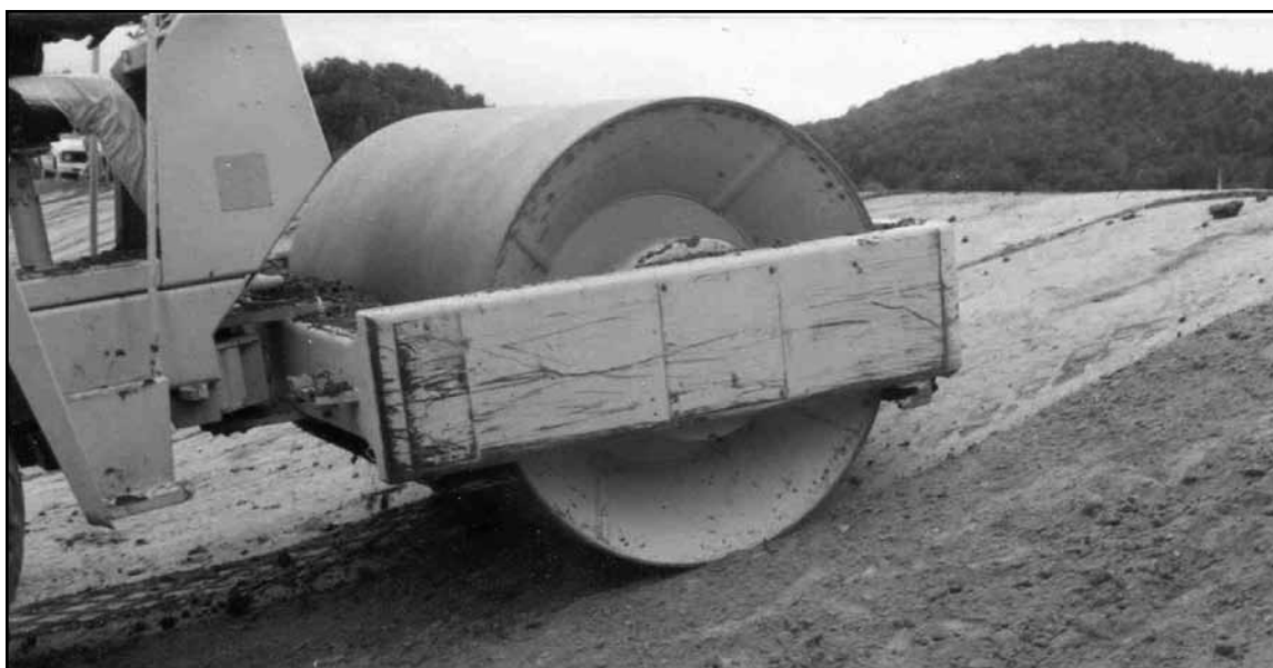
Figure 4-4. Use of a smooth-drum compactor for subgrade preparation.
