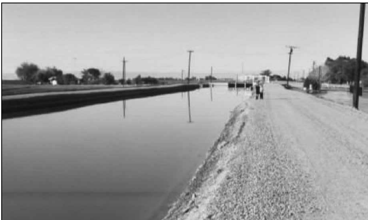
Figure 3-9. Canals present unique design challenges due to the steep sideslopes and the need for continuity of the water supply.
