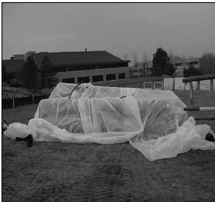
Figure 4-3. Proper storage of Bentomat CL on site.
