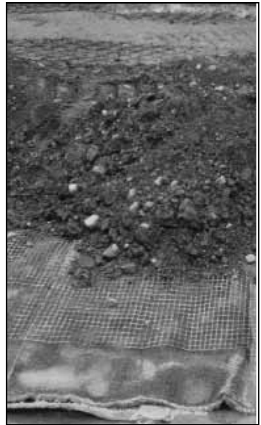
Figure 3-6. A drainage geocomposite was placed below the liner and a geogrid above it to facilitate installation and drainage.
