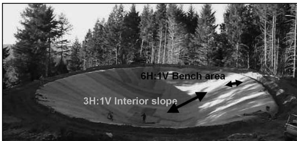
Figure 3-12. A gently sloping bench has several advantages in a decorative pond. m) before a transition to a steeper slope (Figure 3-12). Not only does the bench allow access by wildlife and humans, it serves as a safety device by providing organisms a chance to exit the pond before encountering deep water. A well-designed bench also allows for rip rap (large stone) to be placed for protection against wave action and scouring.
