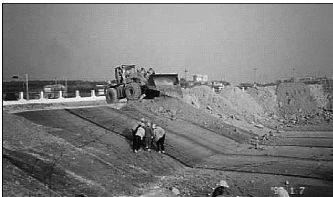
Figure 3-1. Installation of Bentomat CL in a typical wastewater lagoon. Inlet pipes in foreground.
