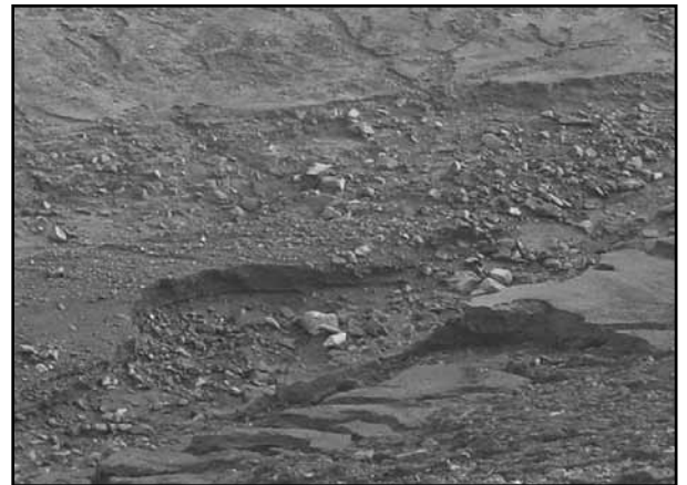
Figure 2-1. Rocky soils may need to be covered with a layer of sand or geotextile prior to liner installation.
