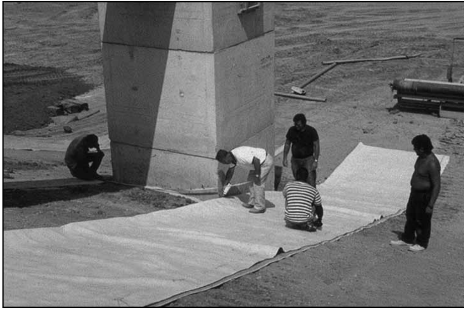
Figure 3-2. Connecting the liner to a manhole in a wastewater treatment lagoon.
