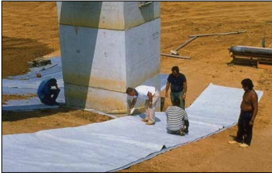
Figure 3-2. Connecting the liner to a manhole in a wastewater treatment lagoon.
