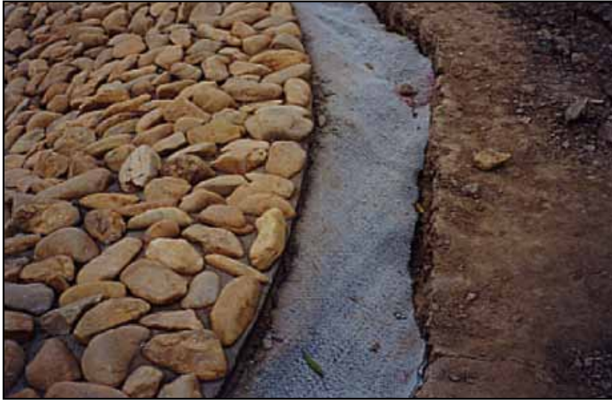
Figure 3-3. In this pond, a layer of cover soil protects the Akwaseal and provides a foundation for a geotextile, upon which large stones are set in mortar. This armored slope will not be subject to erosion or deterioration by people or animals. This technique may not be applicable in freeze/thaw zones.
