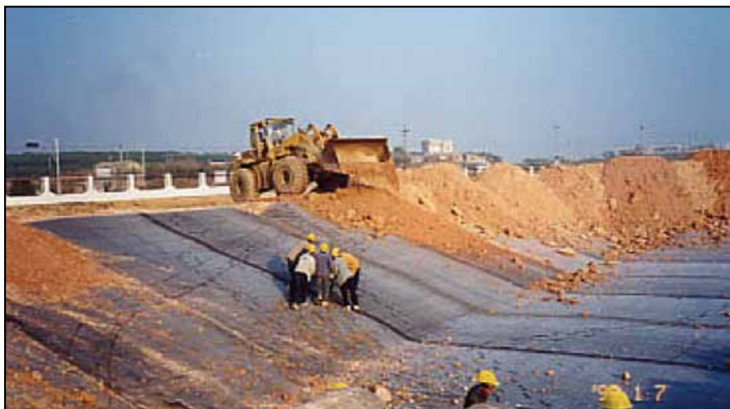
Figure 3-1. Installation of Akwaseal in a typical lagoon. Inlet pipes in foreground.
