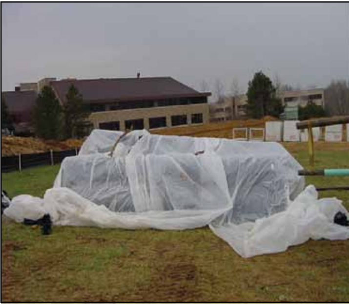
Figure 4-3. Proper storage of Akwaseal on site.
