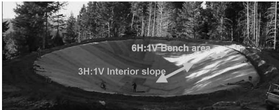
Figure 3-12. A gently sloping bench has several advantages in a decorative pond.
