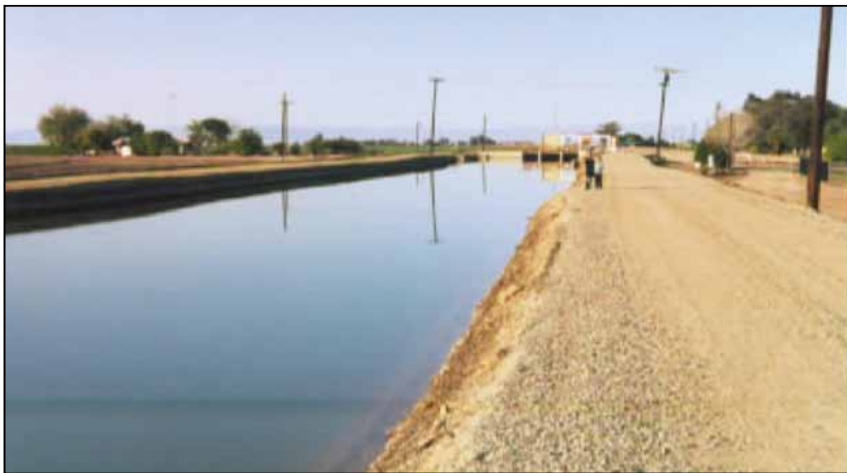
Figure 3-9. Canals present unique design challenges due to the steep sideslopes and the need for continuity of the water supply.
