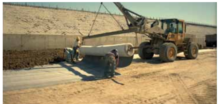
Figure 4-1. Deployment of the liner using core pipe and spreader bar.
