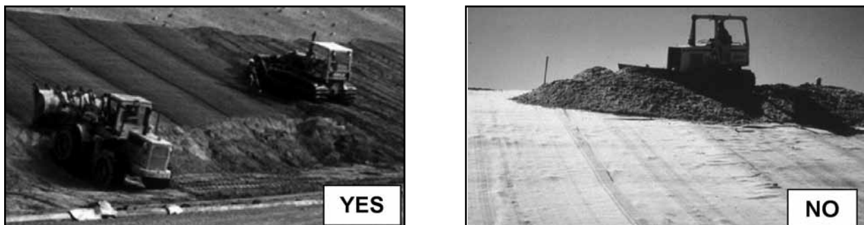
Figure 4-16. Cover soils should be pushed from the bottom of the slope up, not from the top down.
