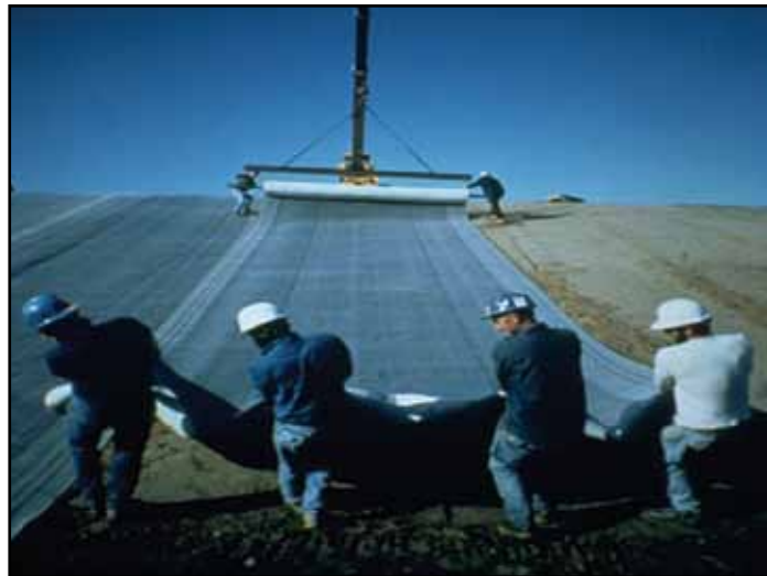
Figure 4-8. Manual deployment down a slope. It is generally not possible to pull the liner upslope.
