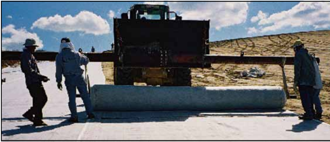
Figure 4-7. Typical means of liner deployment, using a backwards-moving front-end loader.
