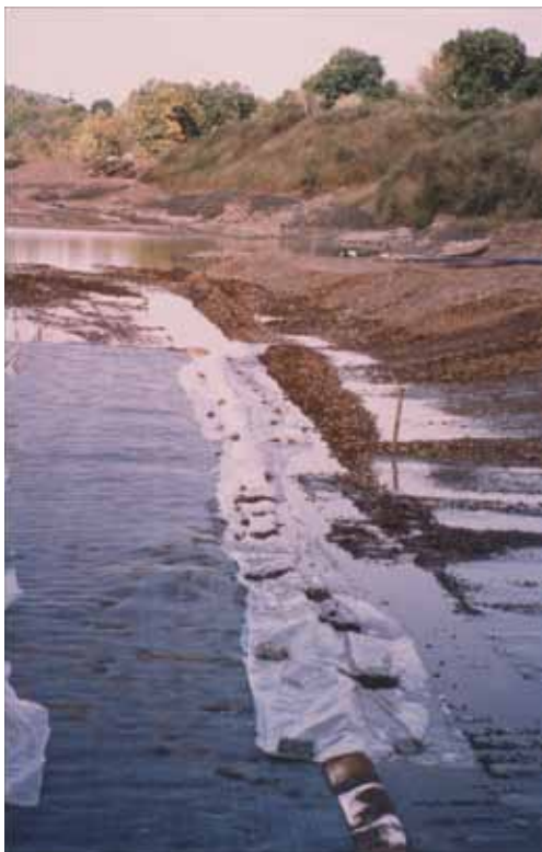
Figure 3-5. High groundwater conditions in wetlands projects make it very difficult to prepare a subgrade and install liner.
