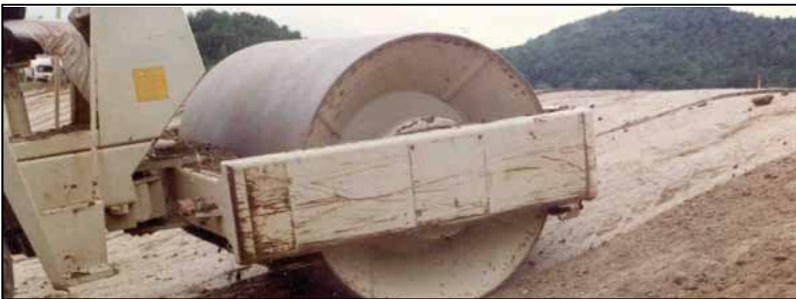
Figure 4-4. Use of a smooth-drum compactor for subgrade preparation.
