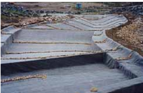
Figure 3-8. Dams help to control water flow and allow saturation of soils behind each dam.
