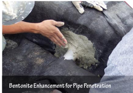
Bentonite Enhancement for Pipe Penetration
