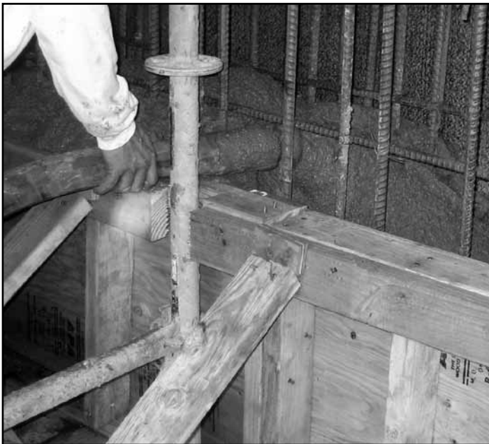
Photo H3-3: SHOTCRETE PLACEMENT IN KICKER FORM
