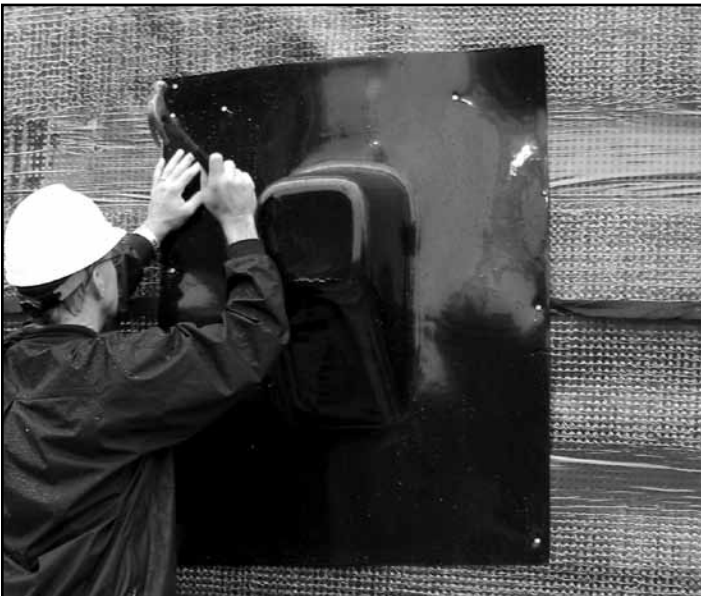
PHOTO 6: TB-BOOT (NON-HYDROSTATIC)
