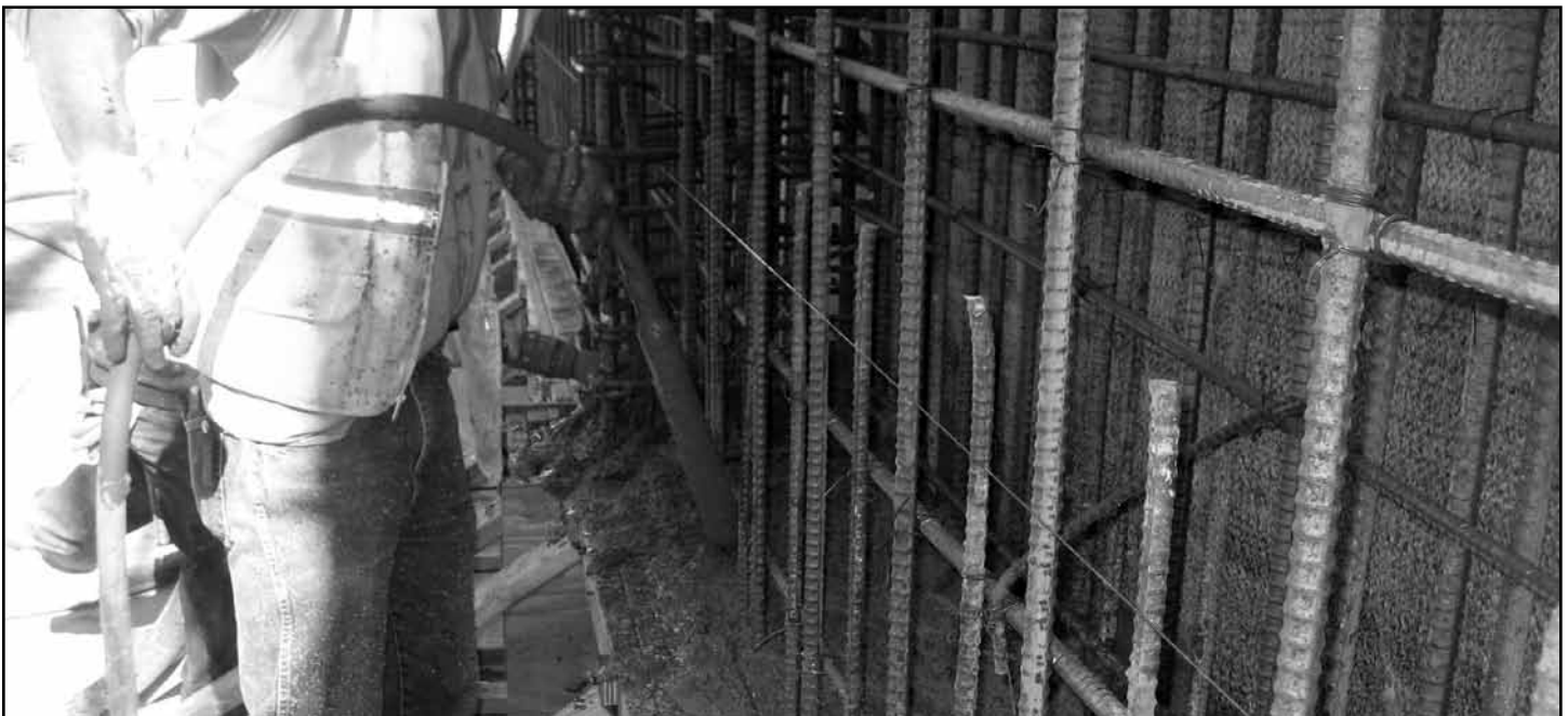
PHOTO 1: KICKER FORM AT BASE OF SHOTCRETE WALL
