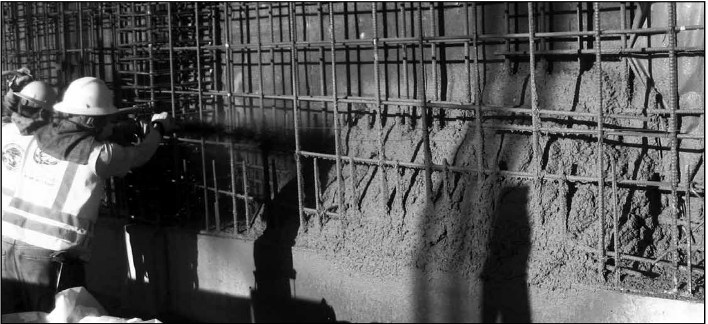
PHOTO 2: SHOTCRETE FOUNDATION WALL
