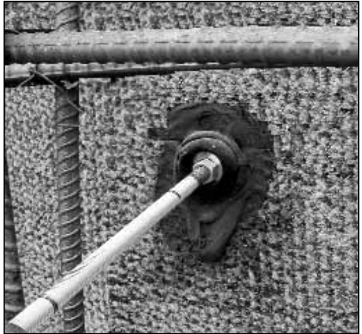
PHOTO 4: REBAR ANCHORAGE DETAILING
