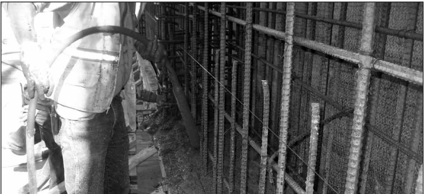
PHOTO 1: KICKER FORM AT BASE OF SHOTCRETE WALL
