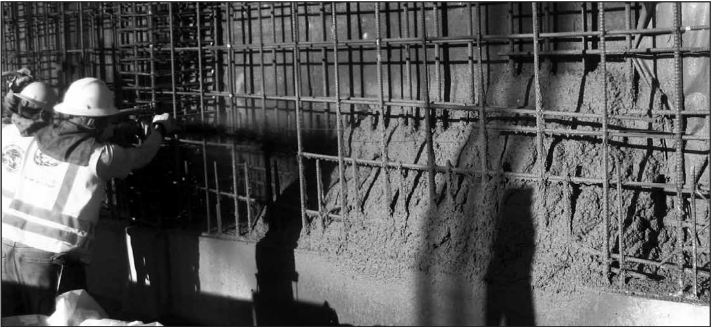
PHOTO 2: SHOTCRETE FOUNDATION WALL
