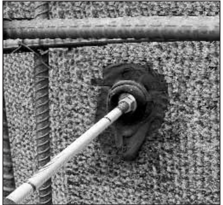
PHOTO 4: REBAR ANCHORAGE DETAILING
