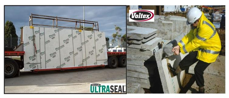
The finished Panel with either VOLTEX, VOLTEX DS or ULTRASEAL SP membranes attached are then ready for transport to site. Once the membrane is attached in this way, it is extremely difficult to remove or damage. If damage does occur a patch of membrane is mechanically fastened over the effected area. If grade levels are not known it is best to leave the membrane at a lower point and mechanically fix it to the height on site.
