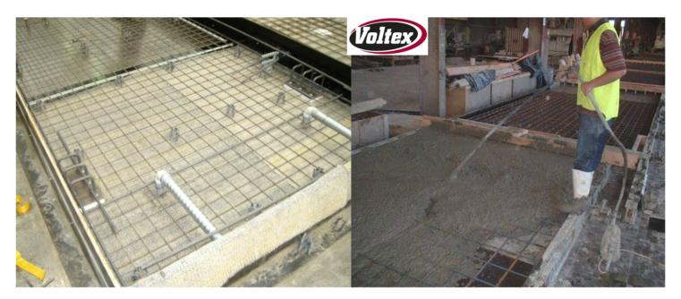
Once the membrane has been installed and detailed, all steelwork is installed as per normal. Concreting pouring and vibration continues as is normally carried out. There is no need for mould release oils to be placed on the Table when VOLTEX or ULTRASEAL are used.
