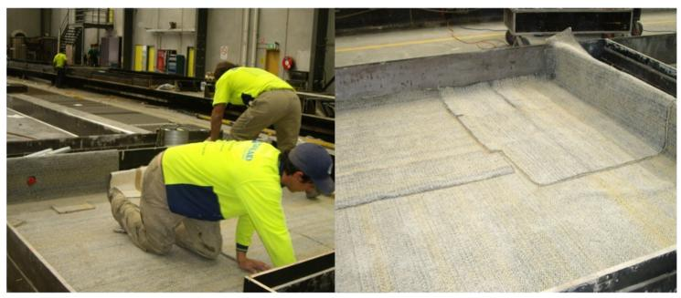
If the membrane is to be placed within the mould VOLTEX, VOLTEX DS or ULTRASEAL SP rolls are placed on the table, cut and fitted to the shape of the Panel. VOLTEX is overlapped on each sheet by 100 mm whilst ULTRASEAL SP is overlapped by a minimum of 50 mm. This operation is usually carried out or overseen by CETCO's Approved Applicators.
