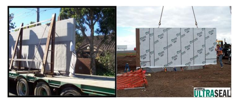
The Panels are lifted into place. The CETCO Approved Applicator should be on site to carry out any detailing or installation of HYDROBAR TUBES should they be required as the Panels are erected.
