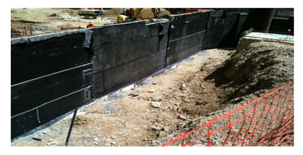
VOLTEX DS installed Panels ready for back-filling operation.
