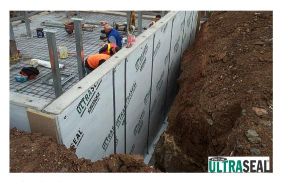
ULTRASEAL SP INSTALLED Panels are shown with Plyboard placed at Panel Joint and overlap on to footing with HYDROBAR TUBES beneath membrane.
