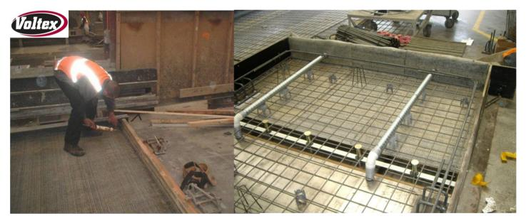
Corners are usually sealed or held in place using CETSEAL. Grouting tubes or penetrations are cut around and sealed using BENTOSEAL. If a termination or grade level is at a point through the Panel the membrane is simply just installed to that mark.
