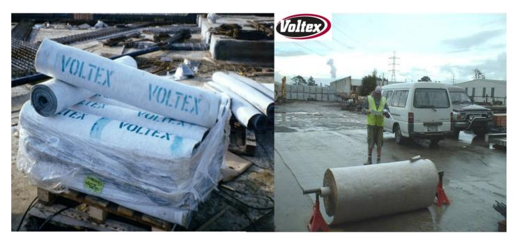
VOLTEX, VOLTEX DS or ULTRASEAL SP rolls are delivered to point of Panel Manufacturing. The VOLTEX range comes in two size rolls: 1.2 m x 5.0 m or 1.66 m x 40.0 m, whilst ULTRASEAL SP is available in 1.2 m x 7.6 m rolls.
