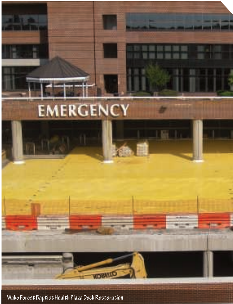
Strataseal HR Hot Rubber Installation
