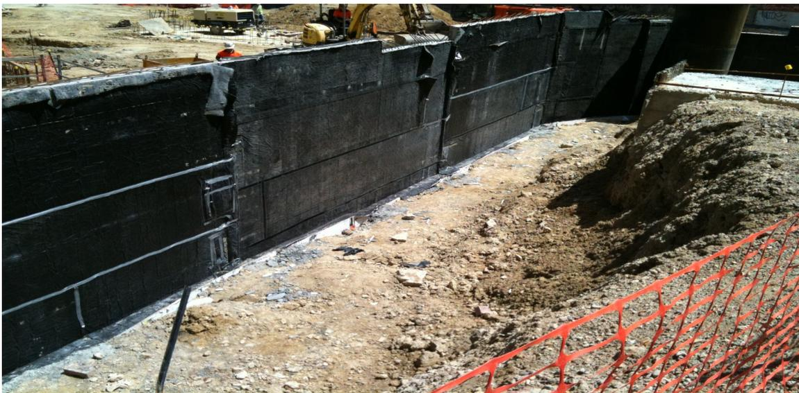
VOLTEX DS installed Panels ready for back-filling operation.
