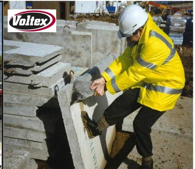
The finished Panel with either VOLTEX, VOLTEX DS or ULTRASEAL SP membranes attached are then ready for transport to site. Once the membrane is attached in this way, it is extremely difficult to remove or damage. If damage does occur a patch of membrane is mechanically fastened over the effected area. If grade levels are not known it is best to leave the membrane at a lower point and mechanically fix it to the height on site.
