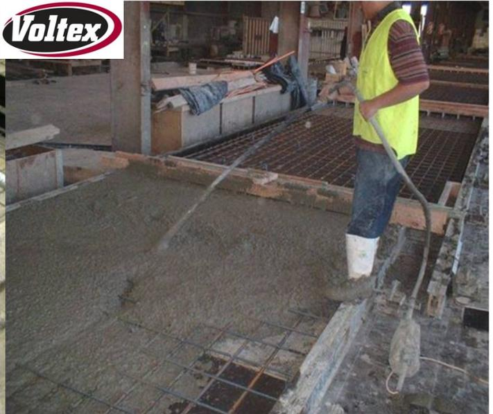
Once the membrane has been installed and detailed, all steelwork is installed as per normal. Concreting pouring and vibration continues as is normally carried out. There is no need for mould release oils to be placed on the Table when VOLTEX or ULTRASEAL are used.
