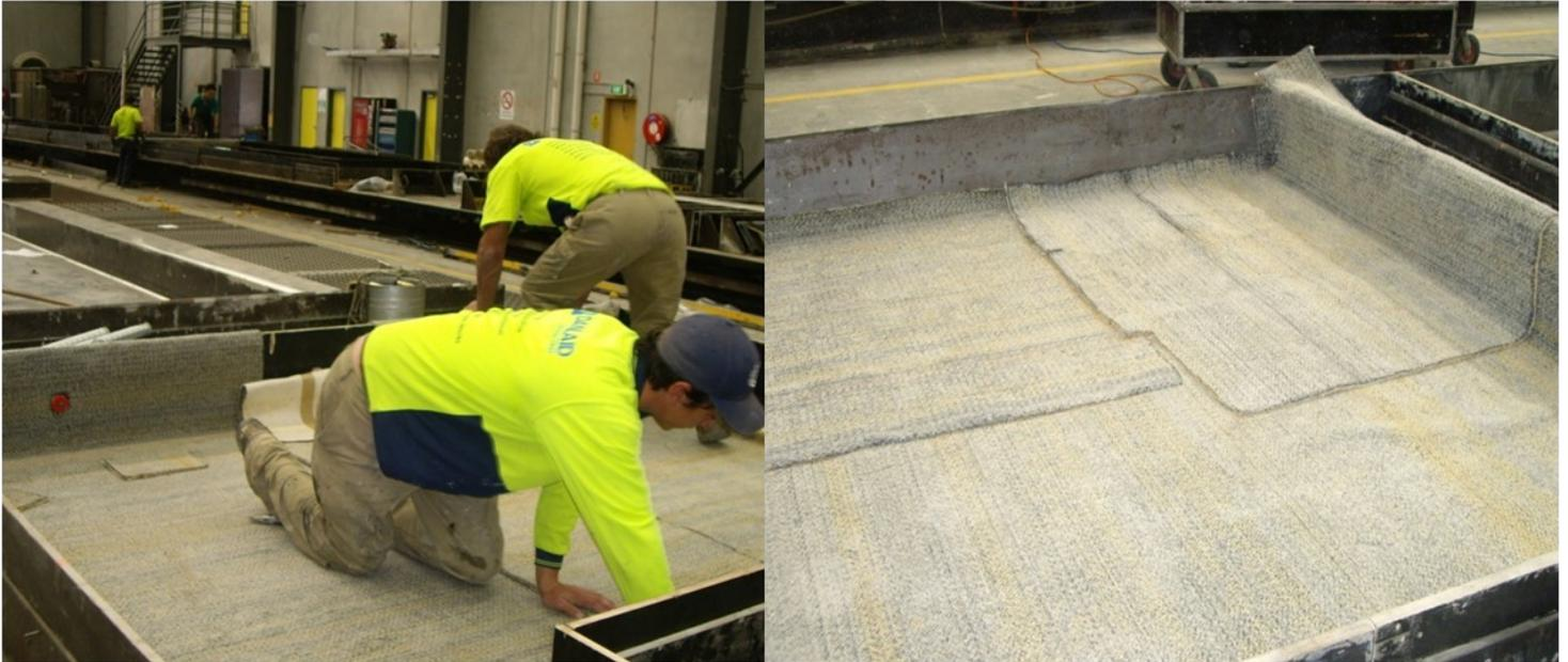
If the membrane is to be placed within the mould VOLTEX, VOLTEX DS or ULTRASEAL SP rolls are placed on the table, cut and fitted to the shape of the Panel. VOLTEX is overlapped on each sheet by 100 mm whilst ULTRASEAL SP is overlapped by a minimum of 50 mm. This operation is usually carried out or overseen by CETCO's Approved Applicators.
