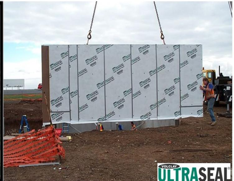
The Panels are lifted into place. The CETCO Approved Applicator should be on site to carry out any detailing or installation of HYDROBAR TUBES should they be required as the Panels are erected.
