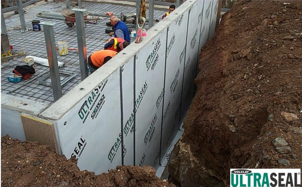
ULTRASEAL SP INSTALLED Panels are shown with Plyboard placed at Panel Joint and overlap on to footing with HYDROBAR TUBES beneath membrane.
