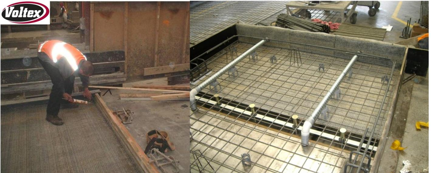
Corners are usually sealed or held in place using CETSEAL. Grouting tubes or penetrations are cut around and sealed using BENTOSEAL. If a termination or grade level is at a point through the Panel the membrane is simply just installed to that mark.
